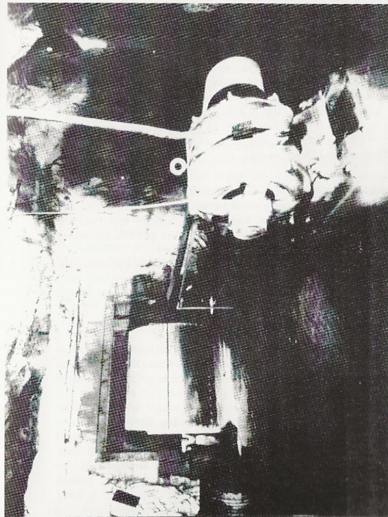
Michigan copper and iron mines were deep and required large ventilation fans to circulate fresh air into the workings. The C&A brought this technology to Bisbee. This fan was installed on the 1,600 level of the Campbell shaft by the C&A to insure adequate ventilation.
