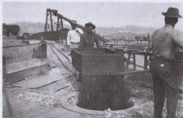
Charging coal to shaft kilns - 1930s
